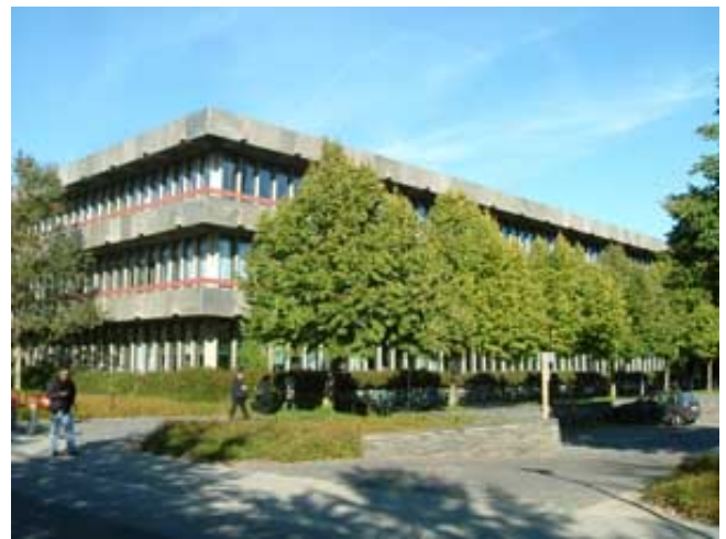
The premises of Technical University of Denmark
