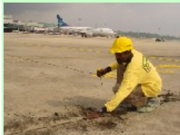
Chipping of the old sealant.
