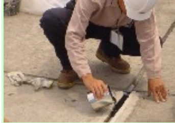
Pouring of the new sealant.
