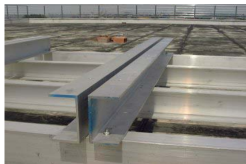
Figure 2. Setting the installation rack on the expansion beam
