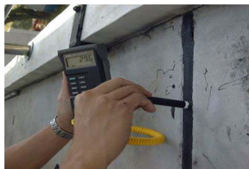
Figure 4. Thermometer to take surface temperature of sealant
