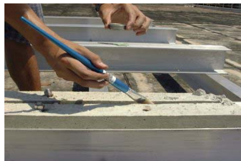
Figure 3. Priming of the concrete substrate
