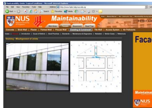
Figure 5. Typical case of staining of metal cladding.
